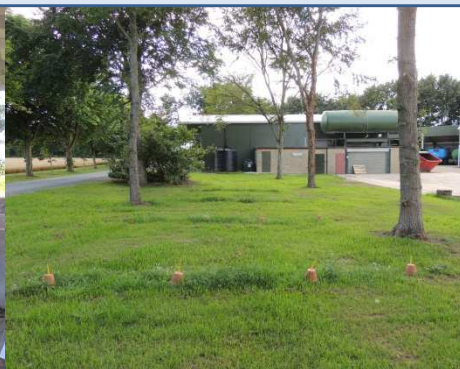
Drain field area with porous pots
