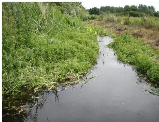
Before and after photographs of the River Tat showing bank re-profiling and redistribution of gravel bed to create a sinuous channel with varied bed levels
