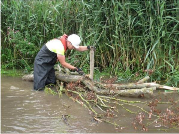
Installing a woody deflector on the River Tat. This helps to provide additional in-stream cover for fish fry and other wildlife.
