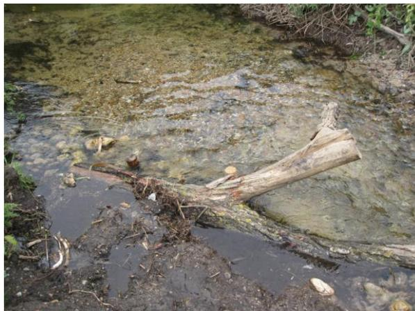
Narrowing the channel using timber. This locally increases flow velocity, mobilising silt and sand to expose the gravel bed.
